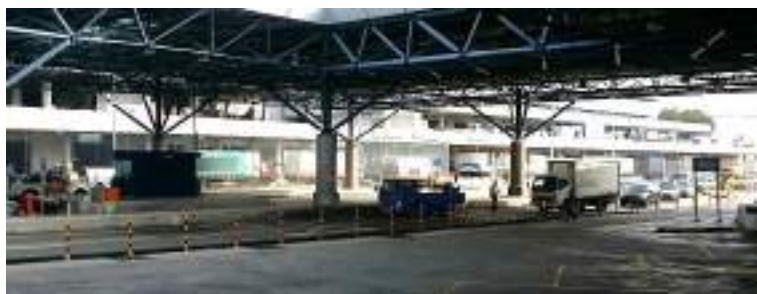
Vehicle stopped at the front end of the checking lane. It created a congestion and stopped free flowing traffic.
